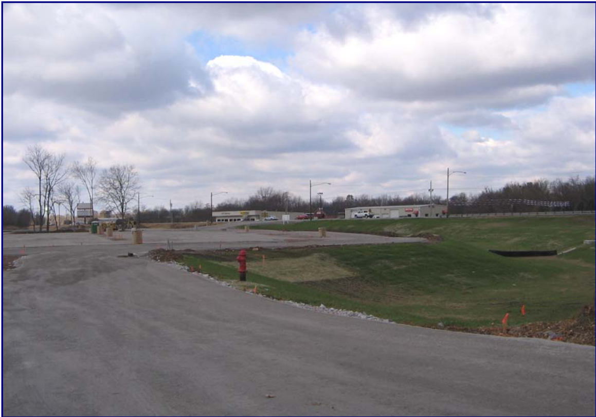
November 22, 2005 – East Entrance of the Lebanon Station
