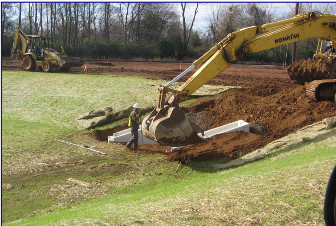
November 30, 2005 – Storm Drainage Work at Donelson Station
