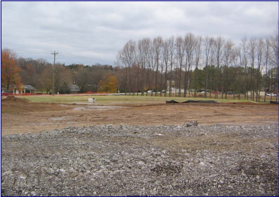
November 23, 2005 – Grading at the Hermitage Station
